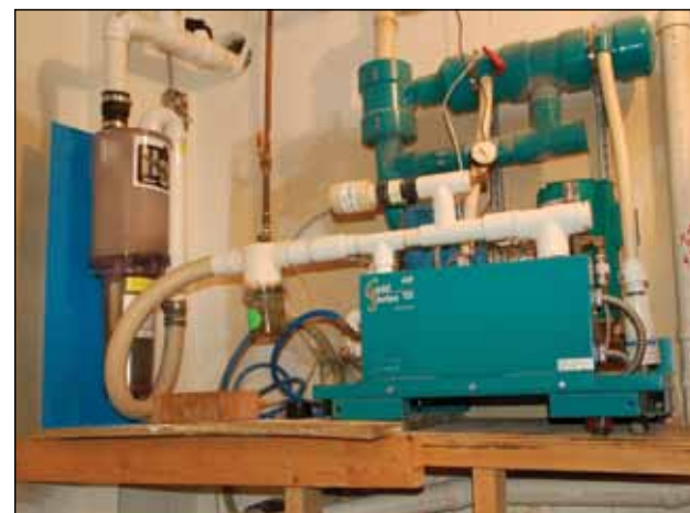
In order to qualify for the Ohio Good DEED program, an ISO 11143 compliant amalgam separator like the Solmetex pictured above must be in use in offices that place or remove amalgam.
